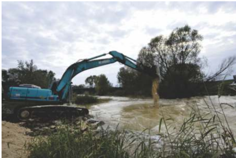
Fig. 15 Gypsum was put into the Torna creek to reduce the pH as Step 1. Ca-nitrate, Mg-nitrate and acetic acid were used downstream in the Marcal river as Step 2. By this way the pH was reduced to about 9 from the original 12-13 before the contaminated water reached the Danube 17
