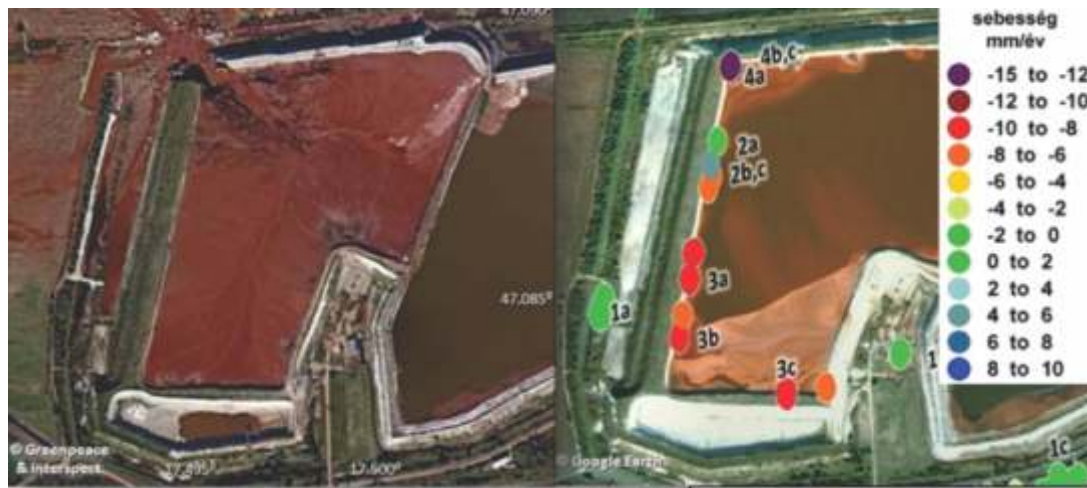
Fig. 18 Sagging of the embankment, March 2003 - August 2010
