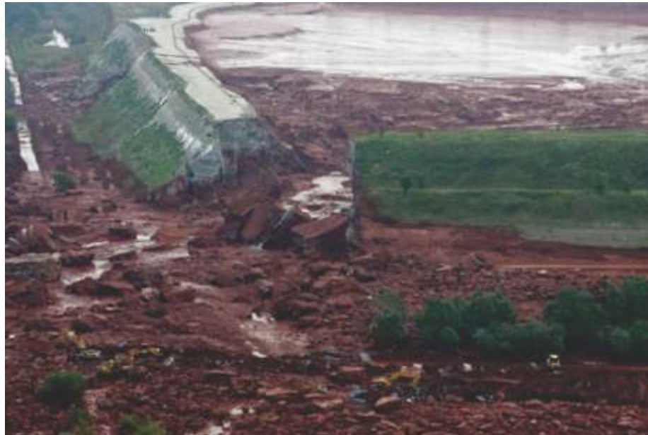
Fig. 13 The ruptured NW corner of the embankment one day after the failure 15 The western edge is almost perfectly vertical.
