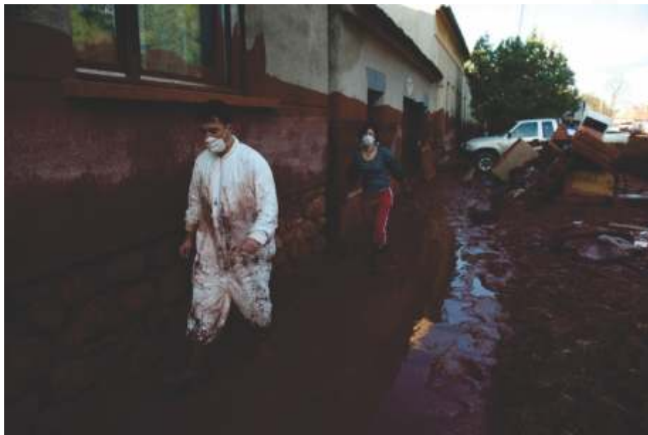
Fig. 9 Affected houses at Kolontár village 11 Traces of a 2 m high red mud sludge wave can be seen
