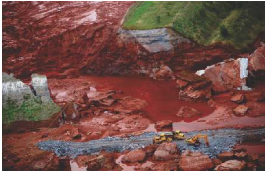
Fig. 14 The affected corner 16 . The upper part of the edge of the western embankment is not contaminated with red mud
