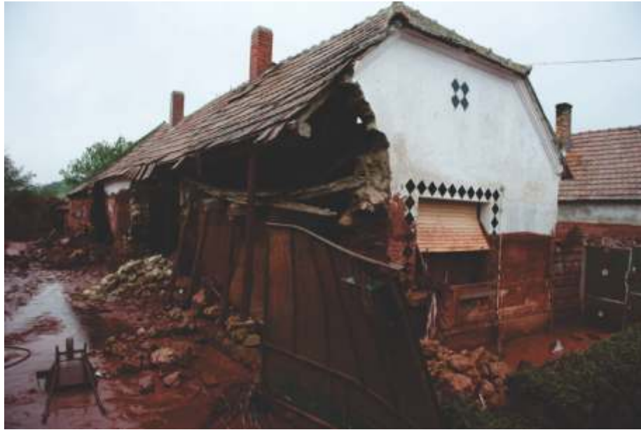
Fig. 8 A badly damaged house made of adobe at Kolontár village 10
